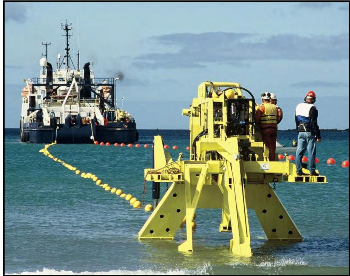
A plough being prepared to start the burial of a cable
